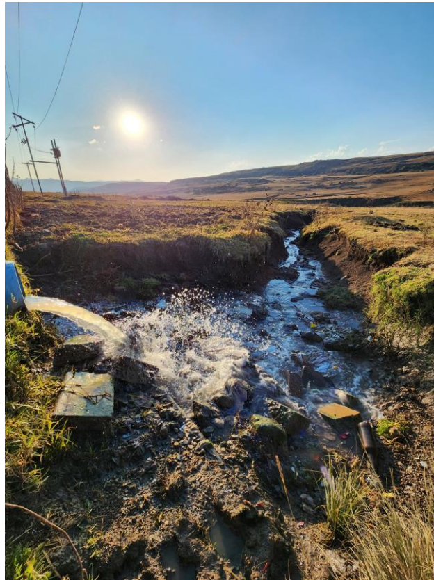
1 - Raw, untreated sewage unsafely discharging from a dysfunctional wastewater treatment works directly into a nearby freshwater stream in the Free State, South Africa. Image credit GroundTruth.
