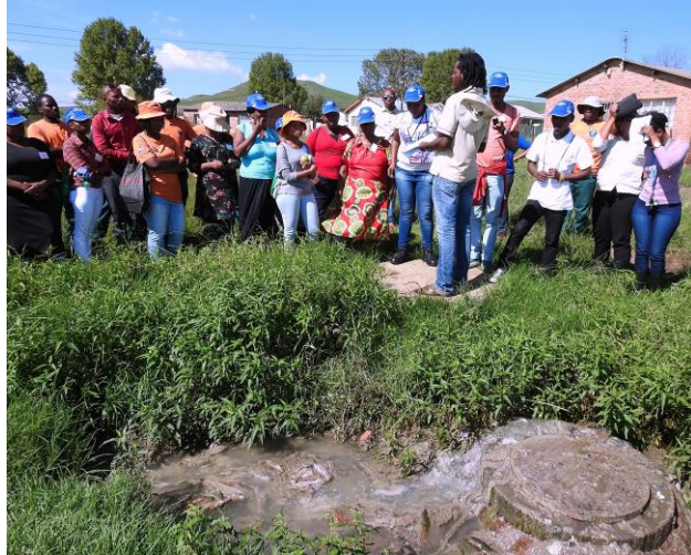
6 - Enviro-Champs discussing the environmental and community impacts of a surcharging sewage manhole in Mpophomeni township in Kwa-Zulu Natal. Image credit the Duzi-uMngeni Conservation Trust (DUCT) and GroundTruth.
