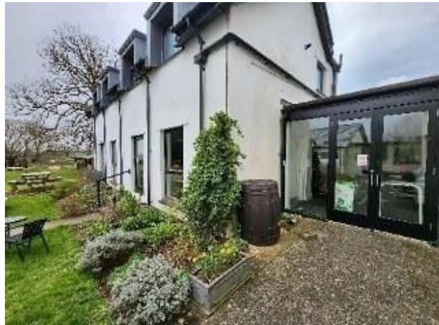
5 - Images of 3 large water butts Installed to service gardens in the Town center. (Picture credit: Great Torrington Water Forum)
